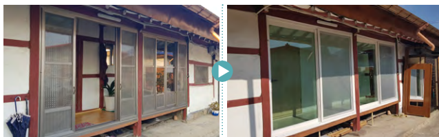
Photo of the house of Guk Jung-gwang before upgrading the windows
